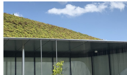
The windows were built in a solar responsive way to reduce glare and heat.
