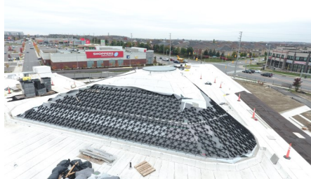
The Georaster elements allow for a stable steep pitched green roof.
