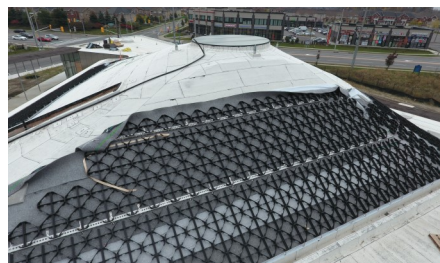
Shear-Fix LF 300 and corresponding TRP Profiles were used as shear barriers.
